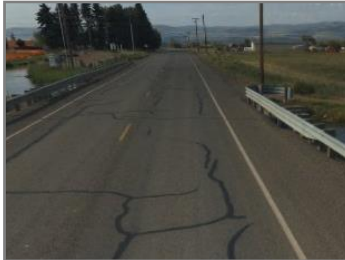
Reecer Creek Rd north of Bender Rd
