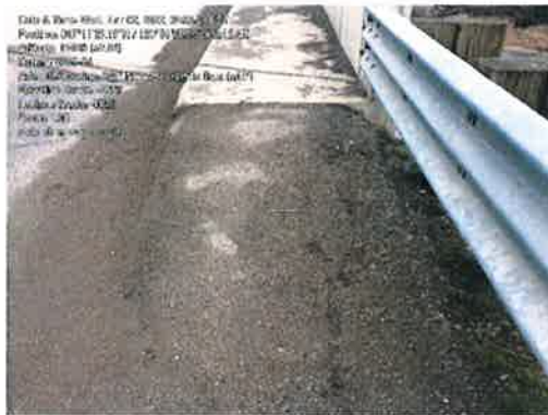
Figures 9 and 10. Examples of Low Compliance (BCR: D) curb ramps at north and south ends of S. Cle Elum Way.
