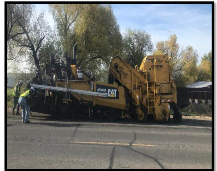
Paving projects maintain infrastructure and safety
