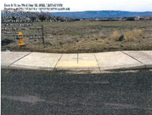
Figures 3 and 4. Examples of fully compliant (BCR: A) curb ramps at Bowers Business Loop and Bowers Rd.
