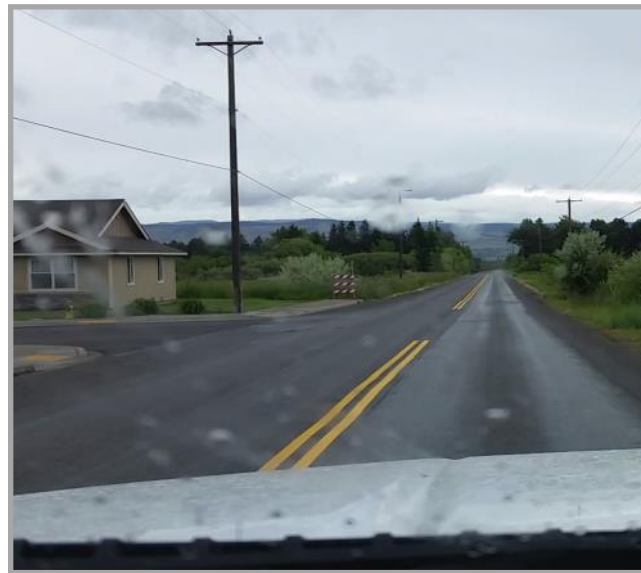
Bender Rd looking west to Reecer Creek
