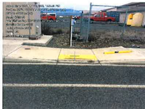
Figures 5 and 6. Examples of nearly compliant (BCR: B) curb ramps at Dry Creek Rd. and Bowers Rd.
