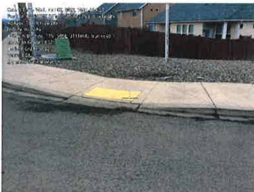
Figures 5 and 6. Examples of nearly compliant (BCR: B) curb ramps at Dry Creek Rd. and Bowers Rd.
