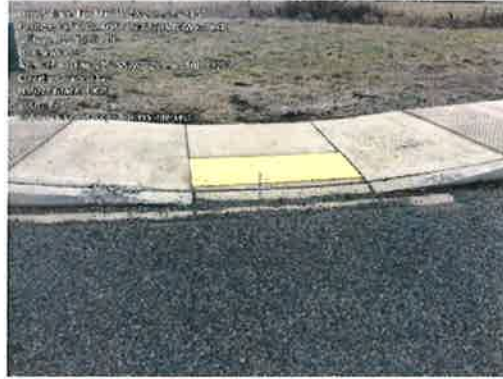
Figures 7 and 8. Examples of Some Compliance (BCR: C) curb ramps at Airport Rd. and Bowers Rd.
