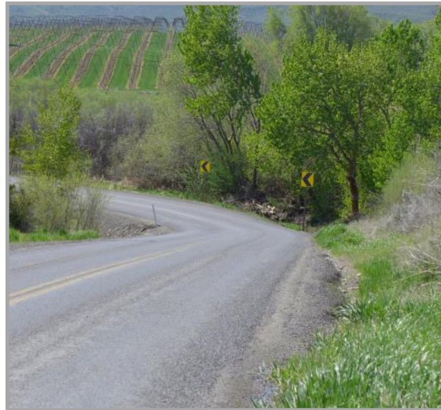
Denmark Rd looking south
