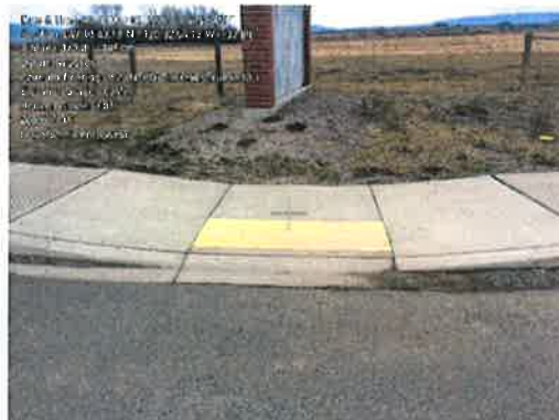
Figures 3 and 4. Examples of fully compliant (BCR: A) curb ramps at Bowers Business Loop and Bowers Rd.
