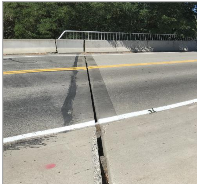
Expansion joint on the S. Cle Elum Bridge
