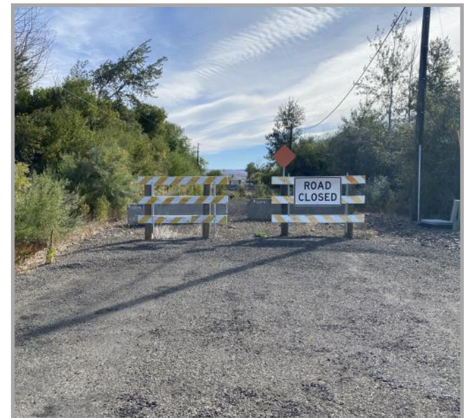
Bar 14 Rd with barricades after bridge removed.
