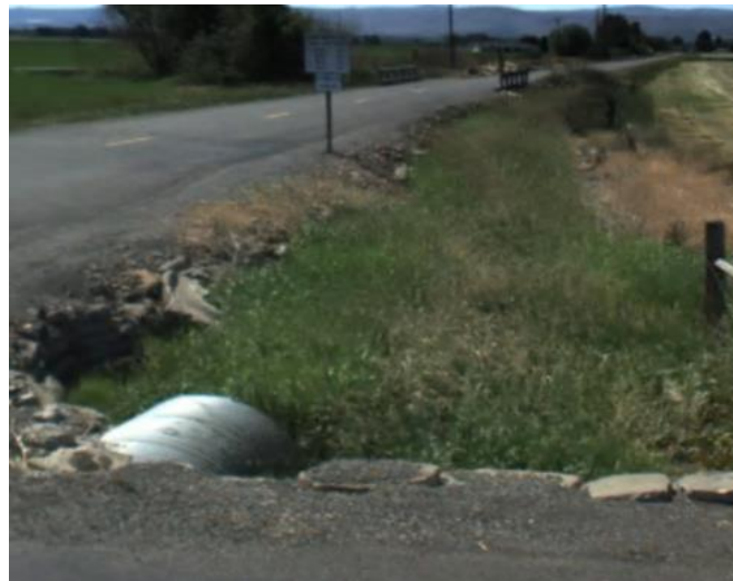
Hungry Junction Rd at Faust Rd culvert
