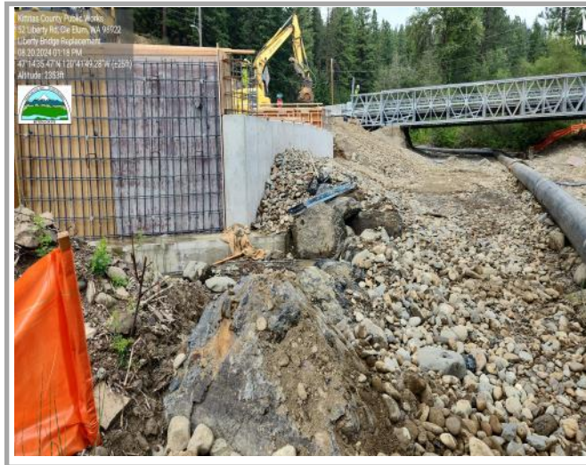
Temporary bridge in distance and new bridge abutments
